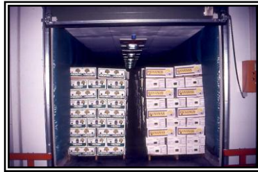
Figure 6: Forced-air ripening room.
